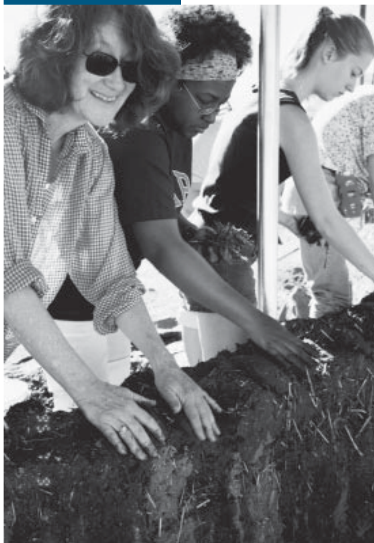
UUSC workcampers mix dirt and straw to make "cob" bricks to build and mold a wall for a day care facility at the Casa de la Misericordia (House of Hope) in Nogales, Mexico, that is scheduled to open in 2004.
